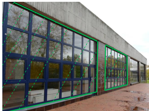
Figure 5. Installing security films [9].
